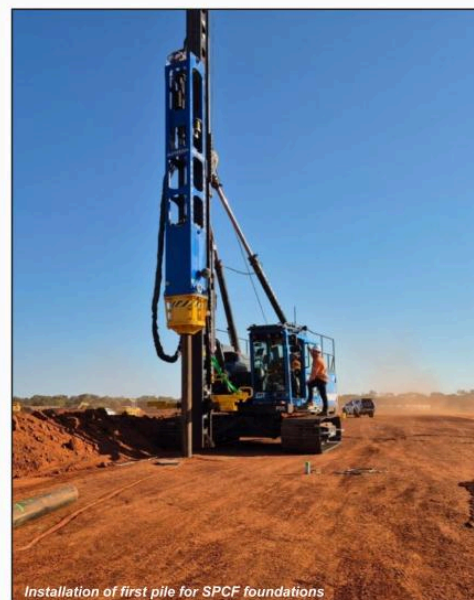
Installation of first pile for SPCF foundations
