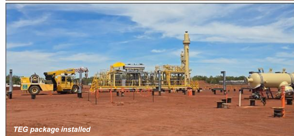
Compressor units installed on SS2 pad
