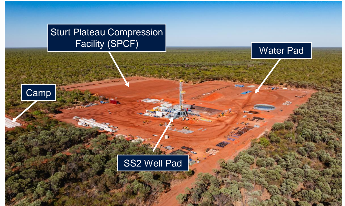
Helmerich & Payne (H&P) super-spec FlexRig® Flex 3 rig on location at 24-hectare SS2 well pad
